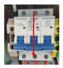
• If there is a PV connection, disconnect the PV by turning the DC switch to off position.
