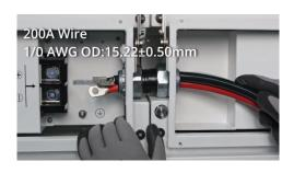
6) Tighten the power cables to the terminals and connect the grounding pole to the SC4-6 copper connection base.
