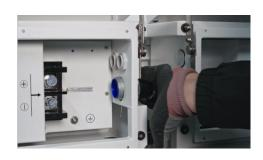
4) Slide the E10 (right) towards the E10 (left) and tighten the conduit with conduit locknut.
